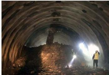
Fig 21. Penetration of the subsea tunnel excavation from both side (Boryeong tunnel, 2019).
