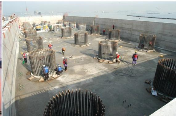
Fig 14. Pylon pile clearance in 2009.
